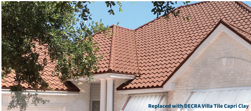
Replaced with DECRA Villa Tile Capri Clay
